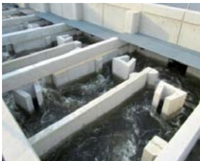
Detail Schlitzpass
